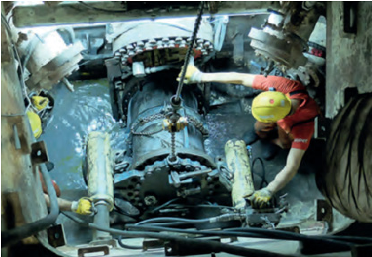
Figure 2. Cutter change within Accessible Cutterhead Spoke in Atmospheric air (Herrenknecht, 2019).
