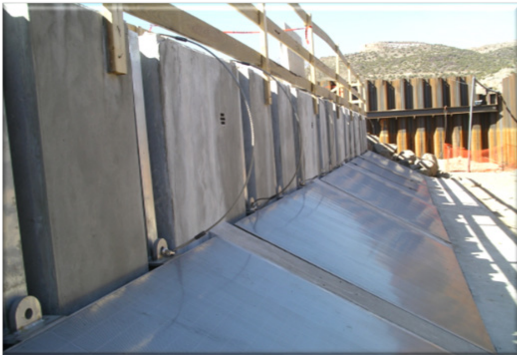
Figure 5. Inclined Flat Plate Screen System at Buckman Diversion
