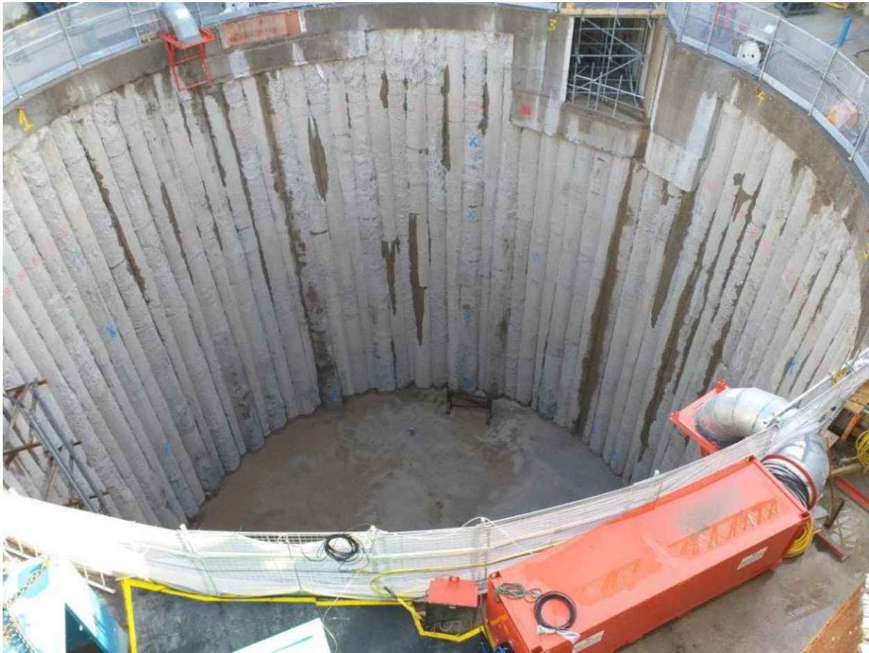
Figure 9. Secant Pile Shaft Thames Tideway Project, UK
