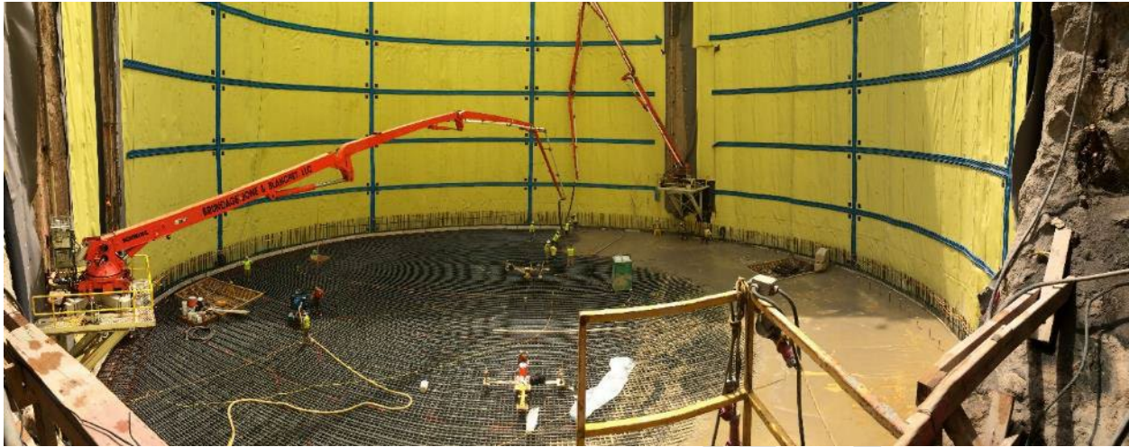
Figure 8. Base Slab Construction for the Blue Plains Dewatering Shaft, Washington, DC
