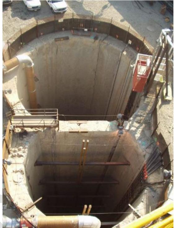
Figure 12. Double-cell Shaft Concept, Northeast Interceptor Sewer in Los Angeles
