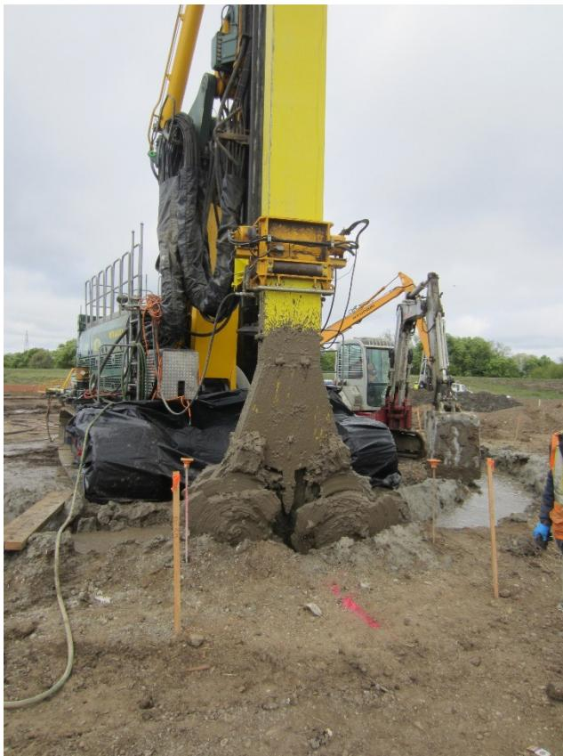
**Figure 3. Deep Mechanical Mixing Rig with Cutters**
