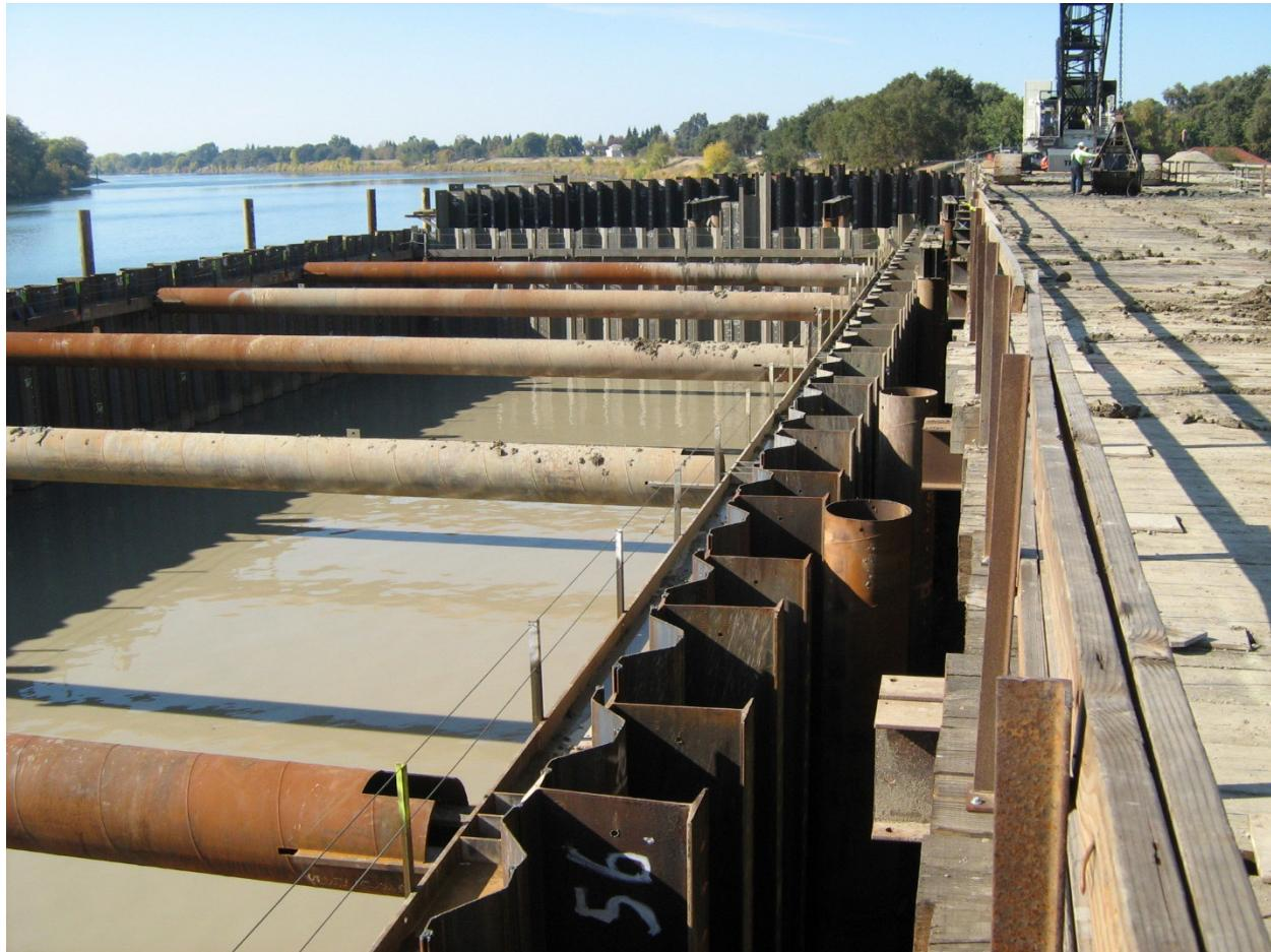
**Figure 1. Cofferdam for Freeport Intake**
