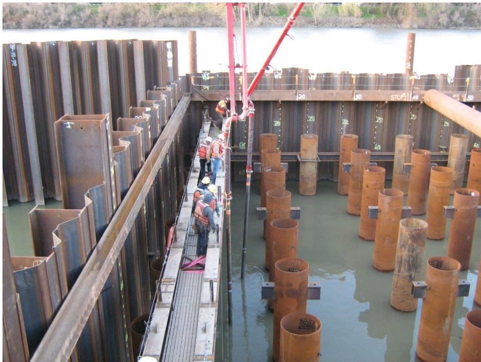
**Figure 4. Tremie Concrete Placement at Freeport Intake**
