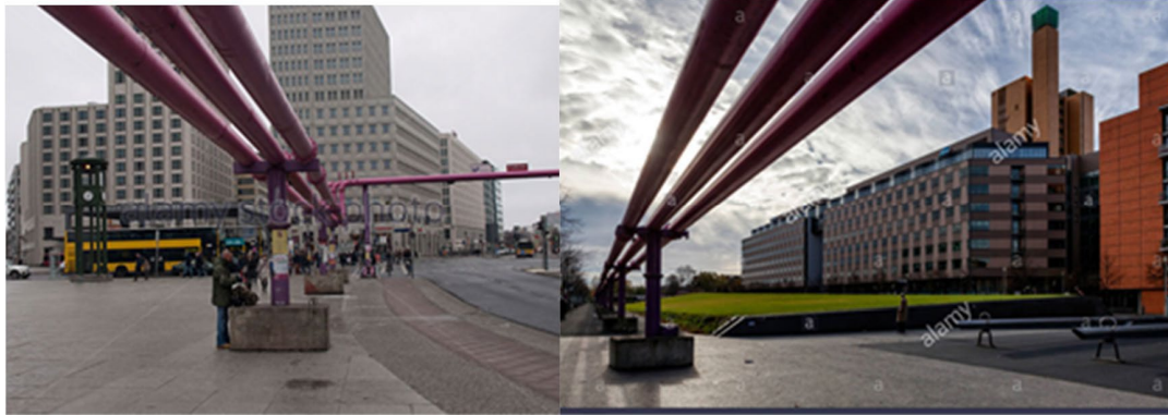
Fig. 5: Elevated slurry lines through Berlin/Germany
